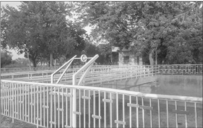
The water tank at Khejarli
